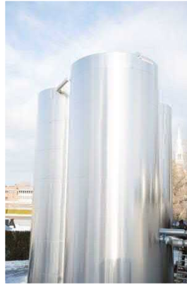
Silos and mechanical room (during installation)
