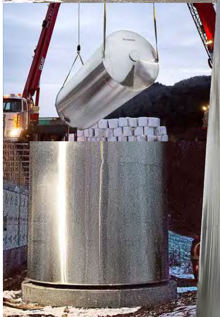
Delivery and installation of a 21,000 Imp. gallons maple sap silo
